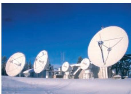
TTC antennae used for the control of the SIRIUS satellites. The antennae are located at the SIRIUS Satellite Control Centre in Esrange, in the far north of Sweden.
